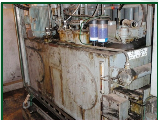
External view of Guillotine 20 Reservoir.
