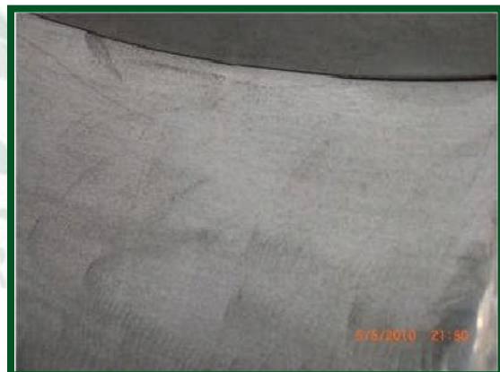
Guillotine 20 Reservoir , 600 USG, after.
