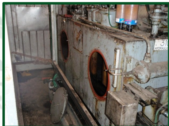
External view of Guillotine 30 Reservoir.
