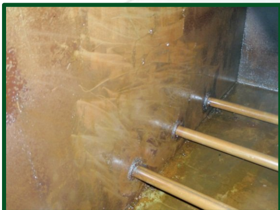
Guillotine 20 Reservoir, 600 USG, before.
