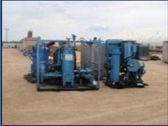
High Velocity Flushing Equipment being staged
