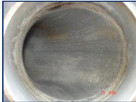
This is an internal view of the pipes, post IAS.
