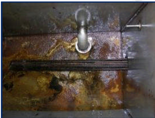
This is an internal view of the reservoir, pre IAS.
