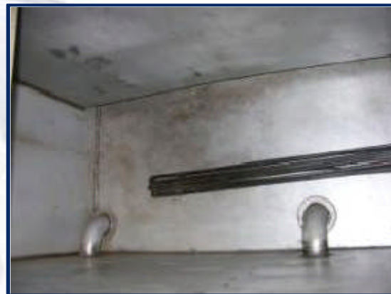
This is an internal view of the reservoir, post IAS.
